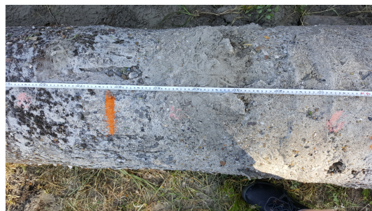
Figure A-3: Photos of diameter changes in pile 8.
