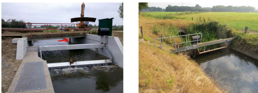
Figure 3.5. Location 2 IJzerbroek weir (108IJZ; main water course, left) and 108TDE weir (tributary, right) in Lage Raam water system, Aa en Maas, near Mill. Red arrow points at measurement location of upstream water level.
