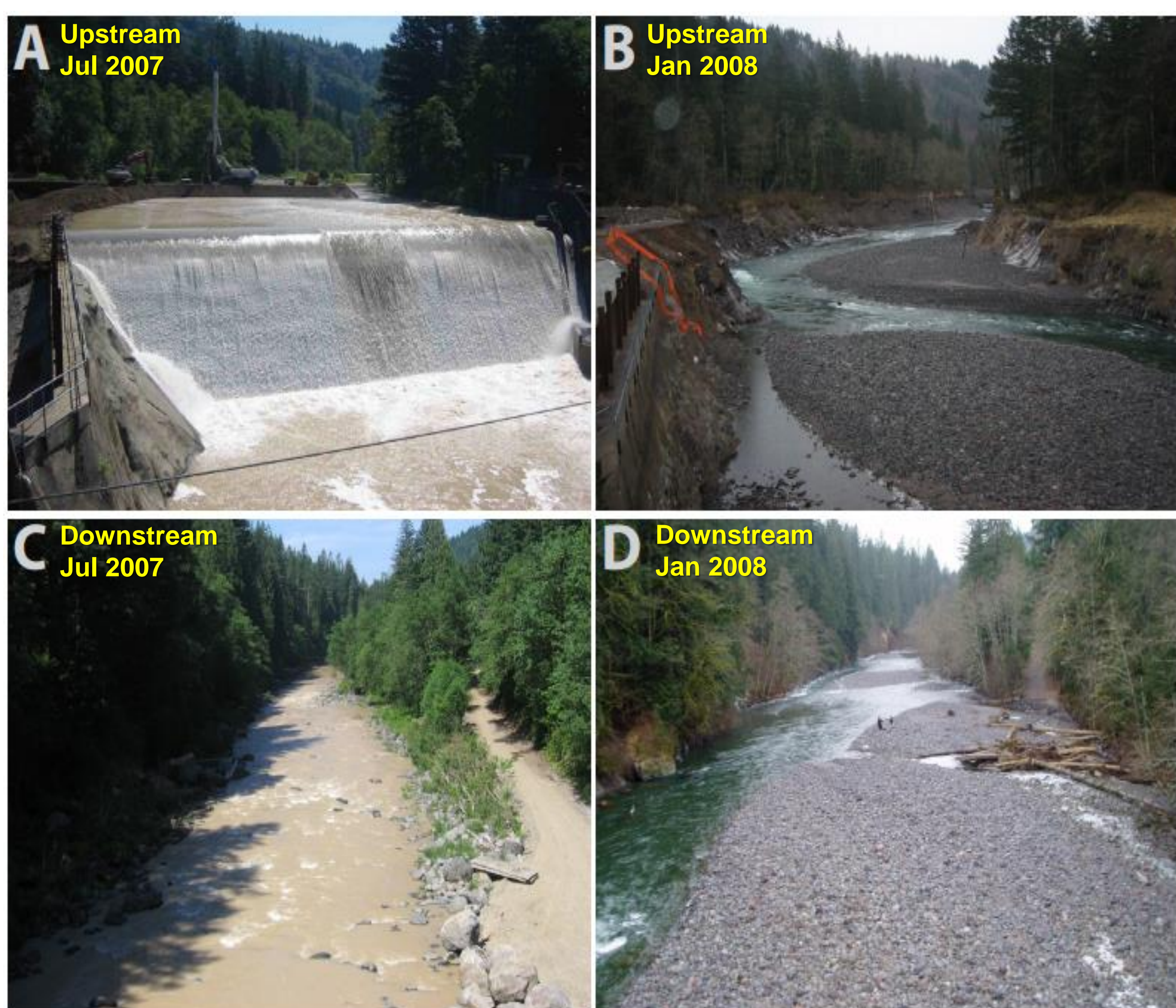
Fig 2. Sandy River before and after Marmot Dam removal (Podolak, 2011).
