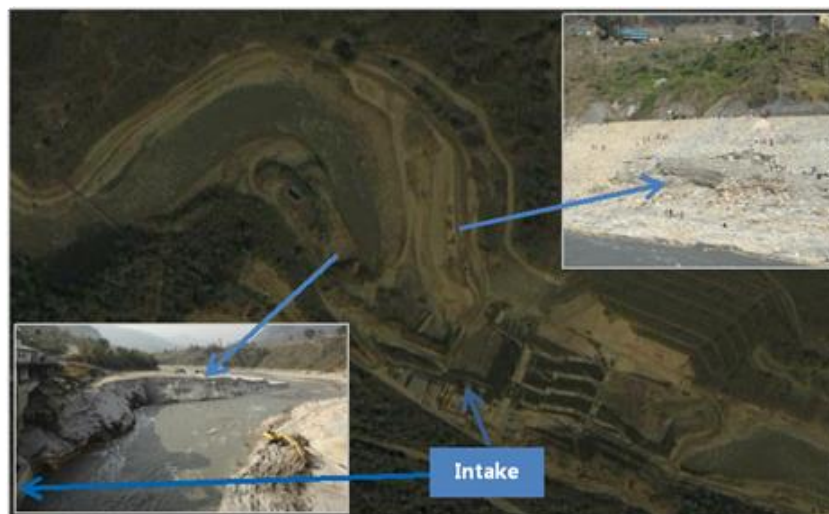
Figure 1. Google earth image of dry Middle Marsyangdi reservoir in Nepal with pictures of inner bend deposition near the intake and toe erosion at outer bend protection near the spillway
