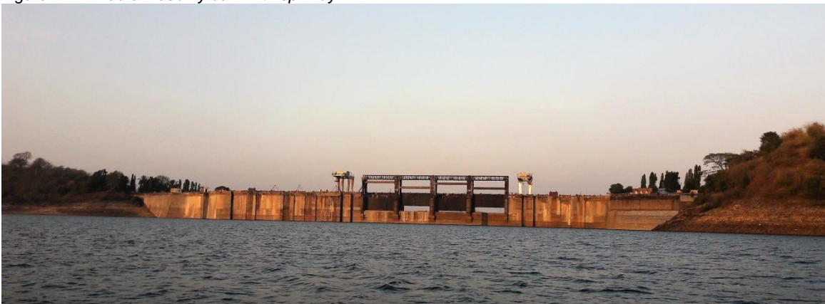
Figure 2.2 Bhadra masonry dam with spillway
