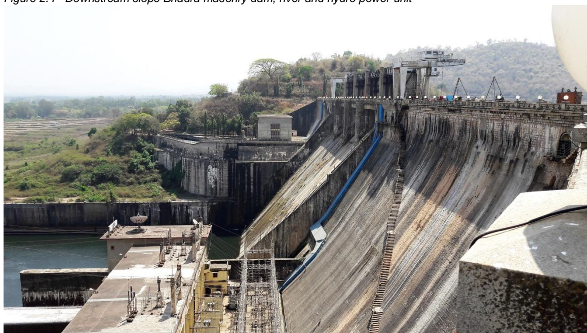
Figure 2.4 Downstream slope Bhadra masonry dam, river and hydro power unit
