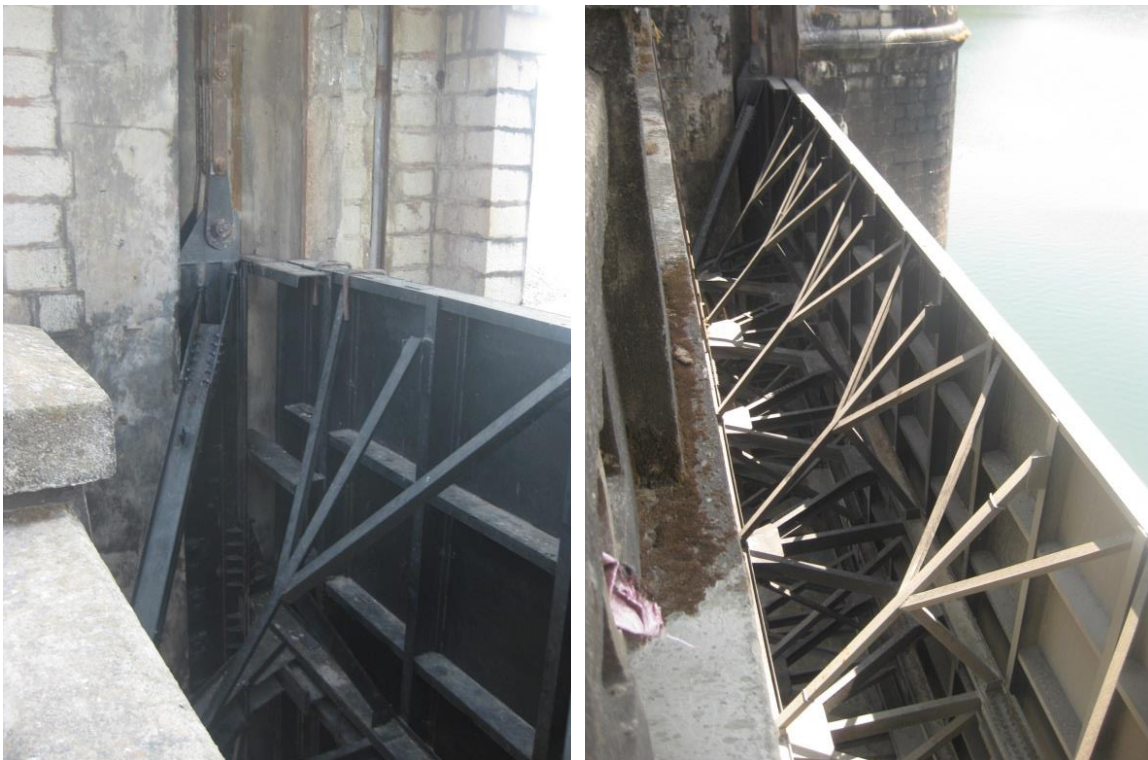
Figure 4.5. View of spillway gates during site visit on 21 February 2017.
