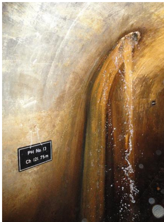
Figure 4.9. Example of drain at main dam and location mark.
