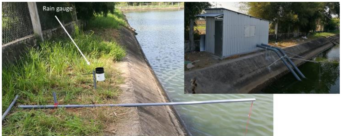
Figure 8-3: Rain gauge installed in TV2 site.
