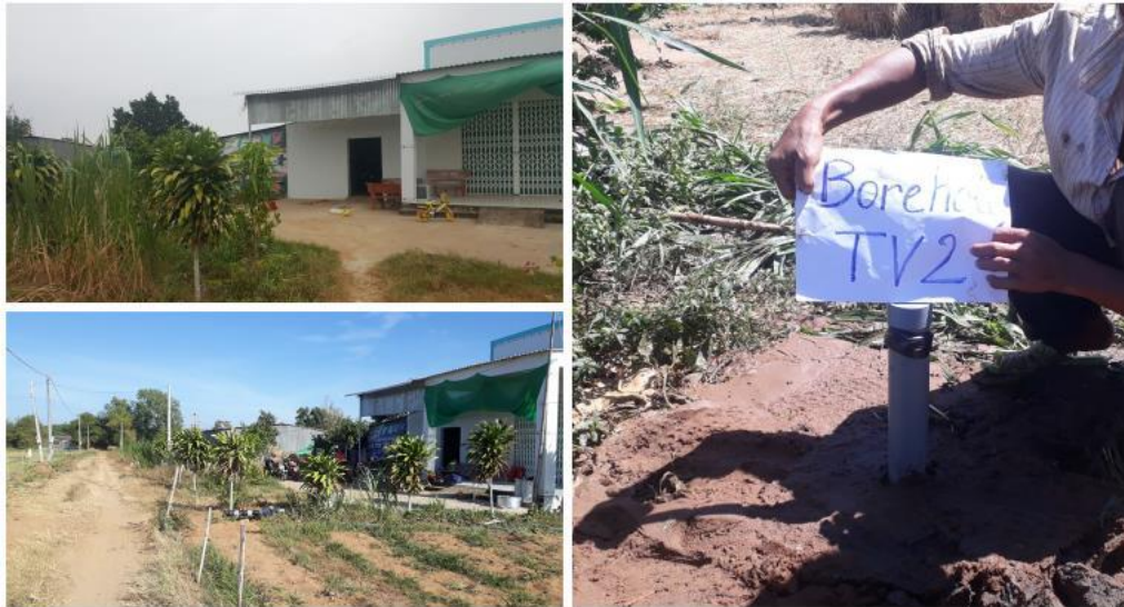
Figure 11-34: Well 2 installed at the TV2 site.
