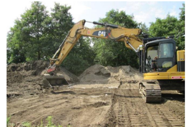
Figure A11.135. Compaction with the excavator shovel only
