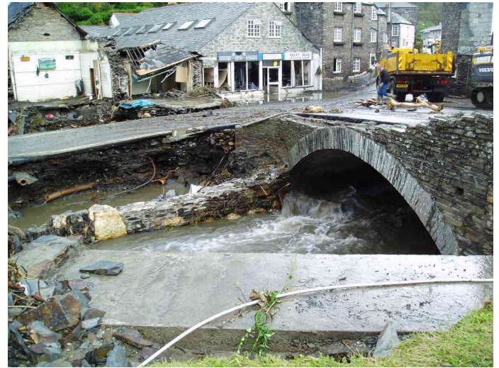
Figure 4 Flash-flood damage at Boscastle (UK), August 2004
