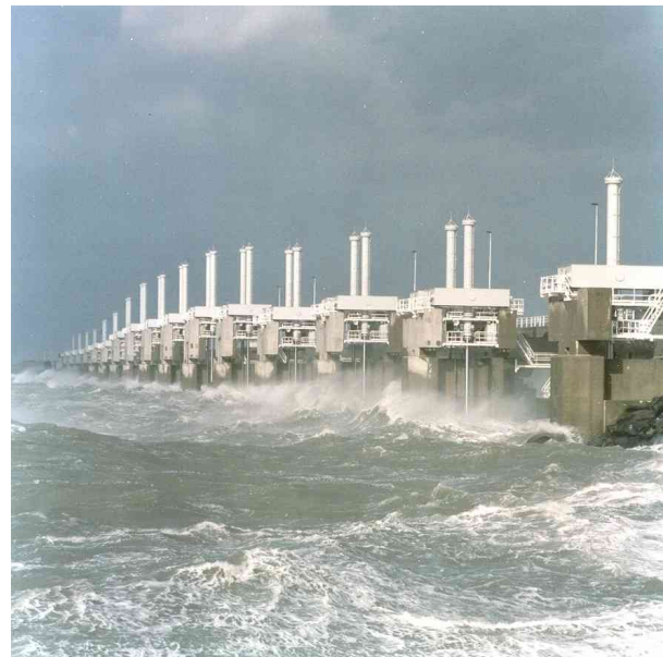
Figure 6 Eastern Scheldt storm surge barrier, the Netherlands
