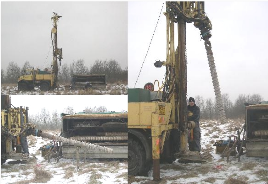
The Århus university crew installing the rick for drilling
