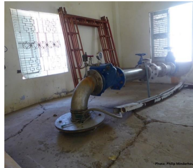
Deeper subsidence, visible by protruding pumping wells
