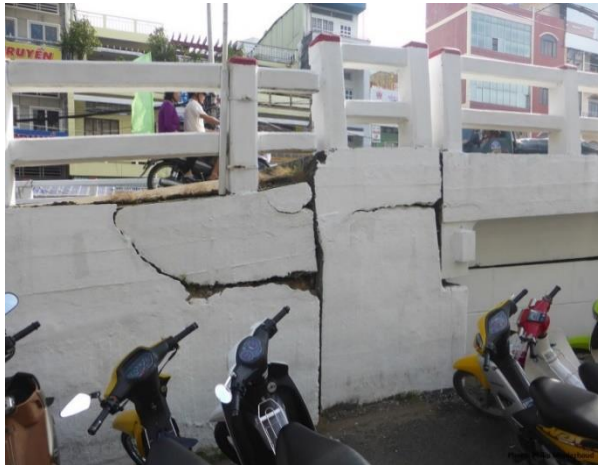
Shallow subsidence, visible around founded bridges and buildings
