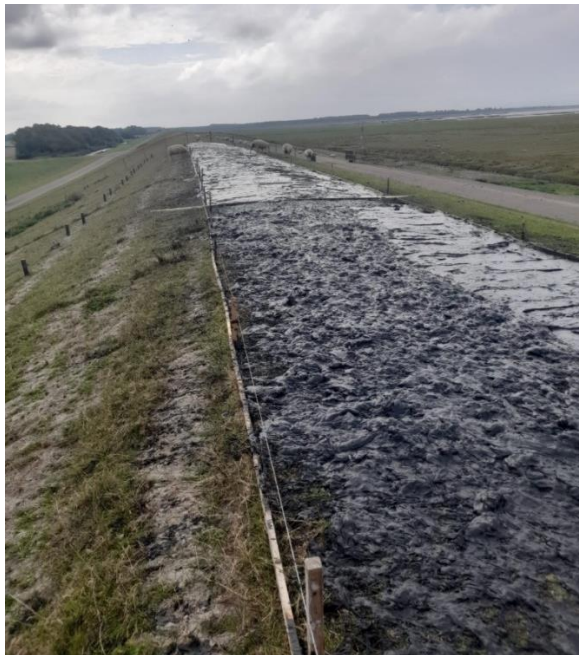
Figure 6.26: Crest of the dike immediately after the application of sediment.
