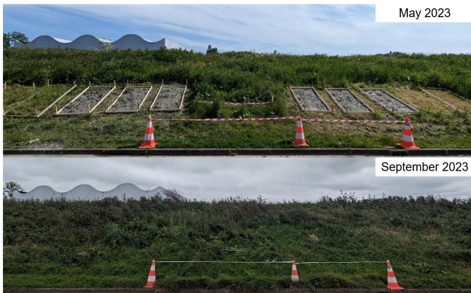
Figure 4.13: Full recovery of vegetation on dike after 4 months.
