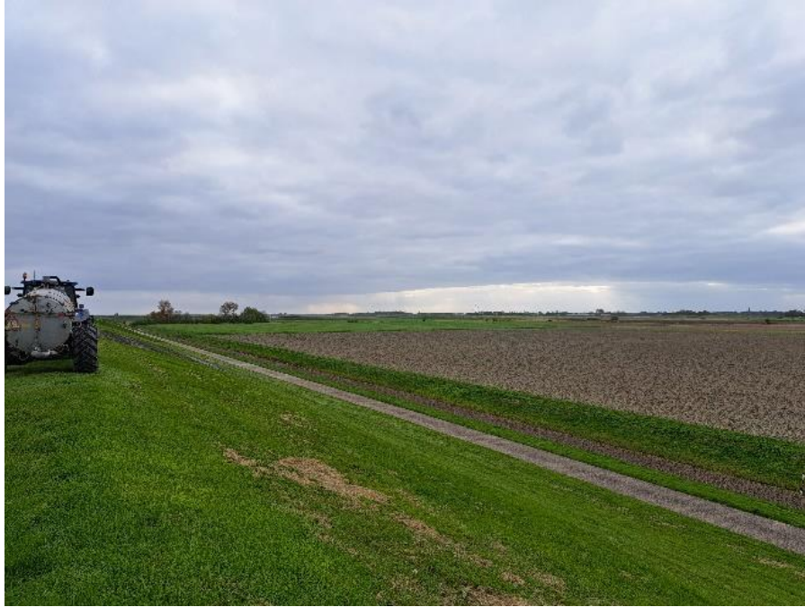
Figure 5.1: Location of the application experiment on the dike which is situated two kilometres to the East compared to the pilot's location.
