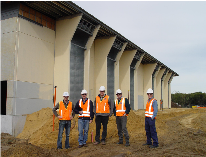
Photo 1: GHD team on site at Perth's largest pump station, Nicholson Road Pump Station
