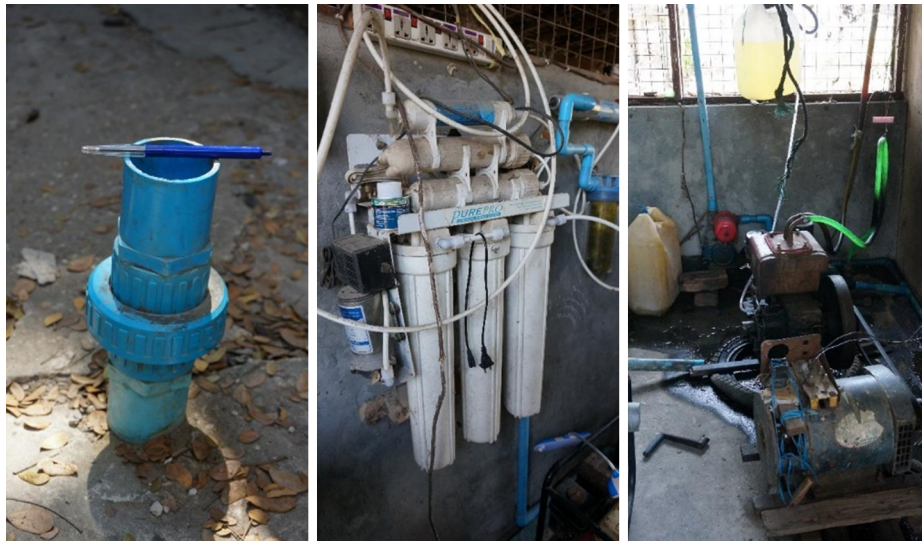
Figure 6a, b, c: actual tube well (a, left). Japanese filtration system (b, middle). Pump (c, right).
