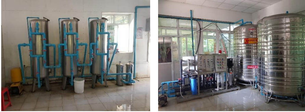
Figure 11a, b: the water filters (a, left). The storage cylinders prior to and after UV treatment (b, right).
