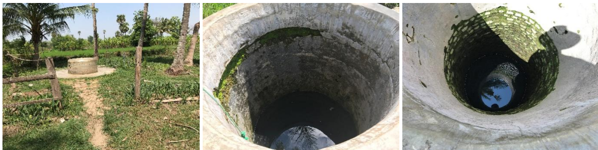
Figure 26a, b, c: the dug well visited in both the rainy season and the dry season (a, left). The SWL during the rainy season (b, middle). The SWL during the dry season (c, right). Photographs courtesy of Jan de Bruin.
