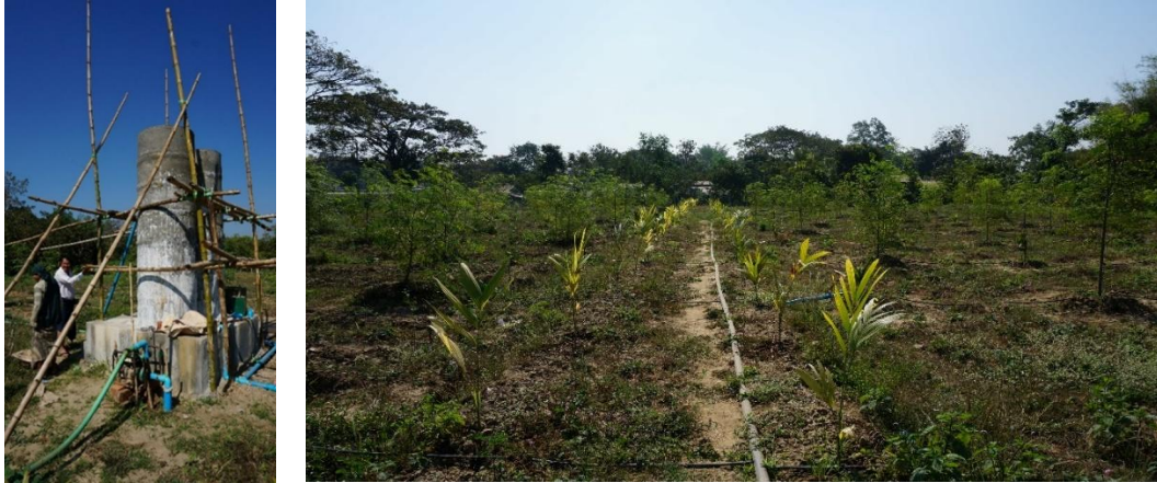
Figure 5a, b: the tube-well with improvised water tower (a, left), which was built to create the pressure needed for the irrigation system (b, right).
