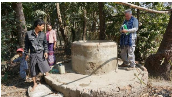
Figure 21a, b: standing next to the first dug well encountered, while the villagers explain its purpose (a, left). The water level is approximately 7 meters below the surface (b, right).
