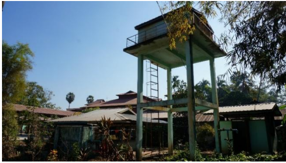
Figure 1a, b: the DRD groundwater well complex, consisting of: the well, the pump house, a water tower and a settling tank (a, left). The pump house contains a diesel fuelled pump (b, right).
