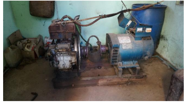
Figure 1a, b: the DRD groundwater well complex, consisting of: the well, the pump house, a water tower and a settling tank (a, left). The pump house contains a diesel fuelled pump (b, right).
