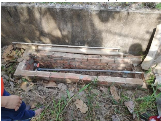
Example of a pump well (location 15 in map 1)
