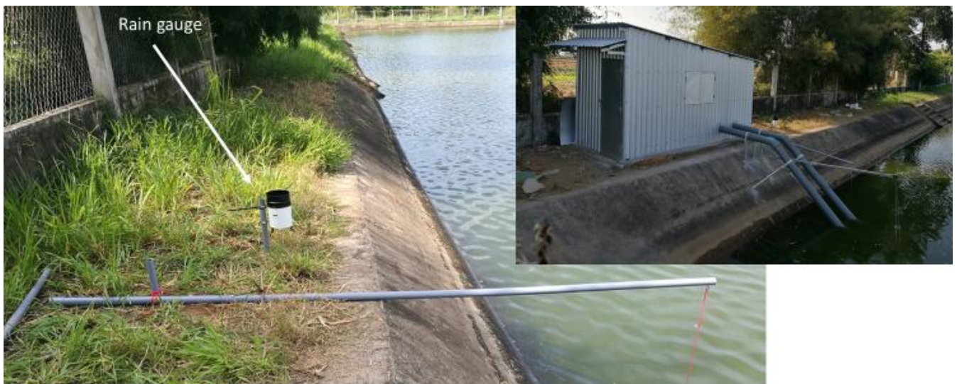
Rain gauge and surface water monitoring installation shown on the left. The photo on the right shows the pumping installation.
