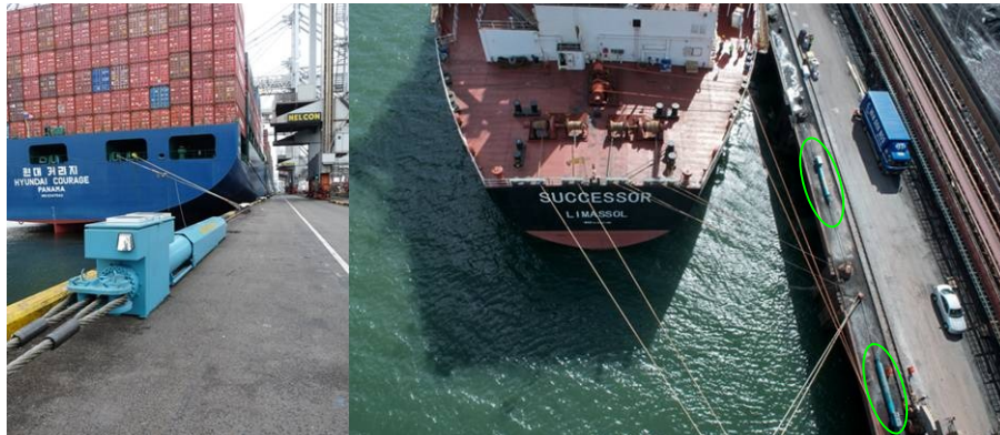
Fig. 3: Example of a recent development in mooring techniques: the Shoretension system (source: www.shoretension.com ).
