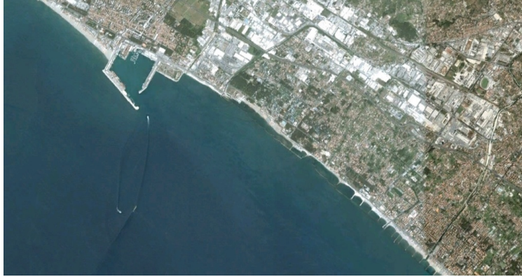
Fig. 7: Port of Carrara, Italy (source: Google Earth). Sediment transport is directed in south-eastern direction. Sand accumulation occurs at the north-western side of the port. The groins on the eastern, downdrift side of the port indicate the area with erosion problems.
